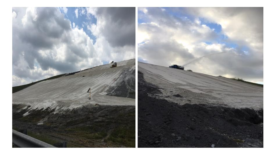
Cell 19 is a 10 Acre ash monofill cell. Work performed while facility is still is active LINER COVER AND PROTECTIVE COVER
