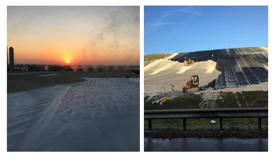
The final cover will consist of the layers from bottom to top with foundation soil, liner or Geomambrane, Geocomposit drainage layer, protective soil and top soil to receive vegetative layer DRAINAGE PIPE INSTALLATION. In Progress Project Cost: \$2.5 Million
